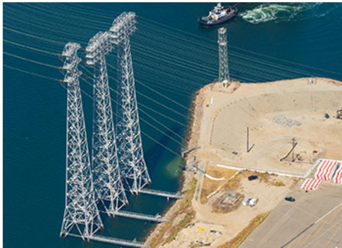
The plans are consistent with the objectives for the Gerald Desmond Bridge Replacement Project. The new bridge will be 205 feet above the Port's Back Channel, while SCE's existing transmission towers' electric lines spanning the Cerritos Channel are only 155 feet above the water. To ensure these electric lines do not impede navigation through the Inner Harbor, the transmission lines and associated towers will need to be raised to at least 205 feet.
