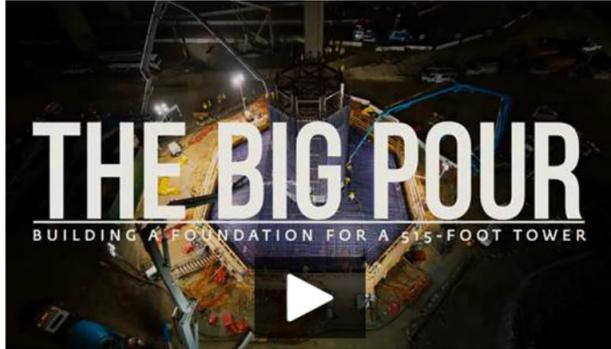
Over **300 truckloads** of concrete were poured in late September for the foundation of one of the two towers that will support the replacement for the Gerald Desmond Bridge.
